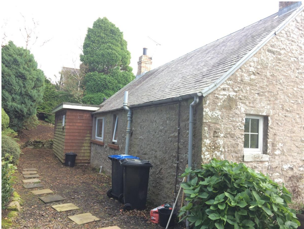
Rear/North Elevation (viewed from West)
