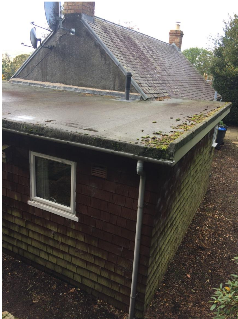
Flat Roof to Original Extension
